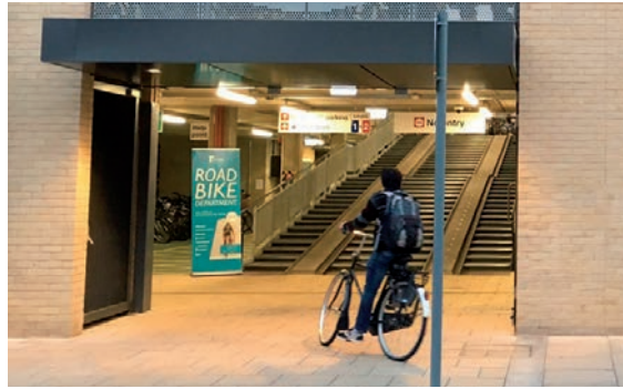
Cycle access to the basement will be via a stepped ramp, plus two cycle lifts
