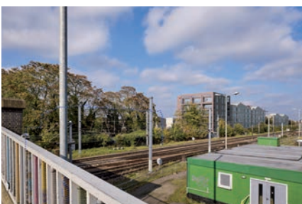
Mill Road Bridge
